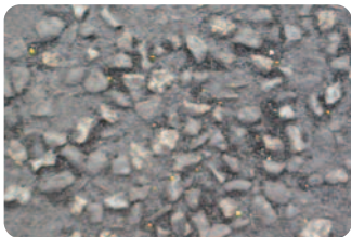
Balgillo Road: Before
